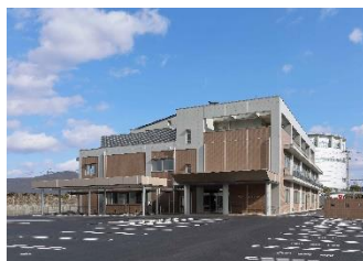
Disability Comprehensive Employment Support Center exterior
